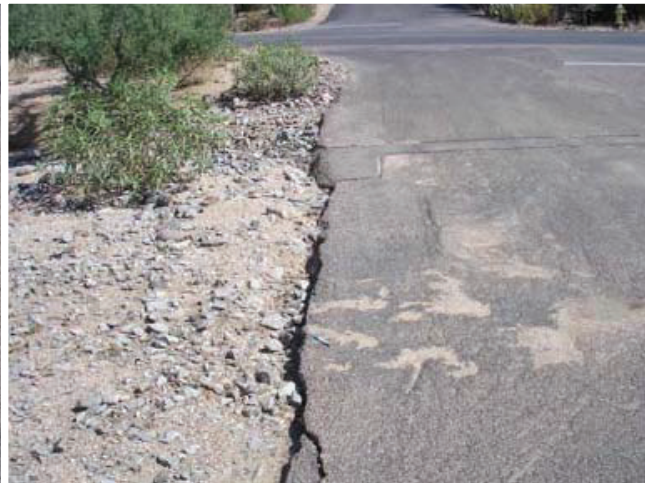
Edge Erosion from Stormwater Runoff
