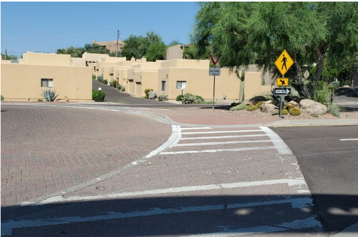
Existing Crosswalk at Traffic Circle on Tom Darlington Drive
